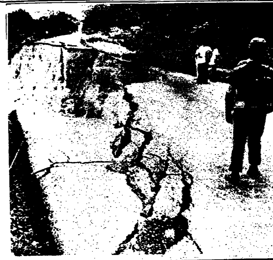
QUAKE HAVOC: A highway leading out of the Venezuelan city of San Cristobal was sheared Sunday by a strong earthquake and slithered down a hillside burying an estimated 35 to 40 homes. Rescue workers found eight dead Monday, but many more victims were believed still buried under tons of earth.
